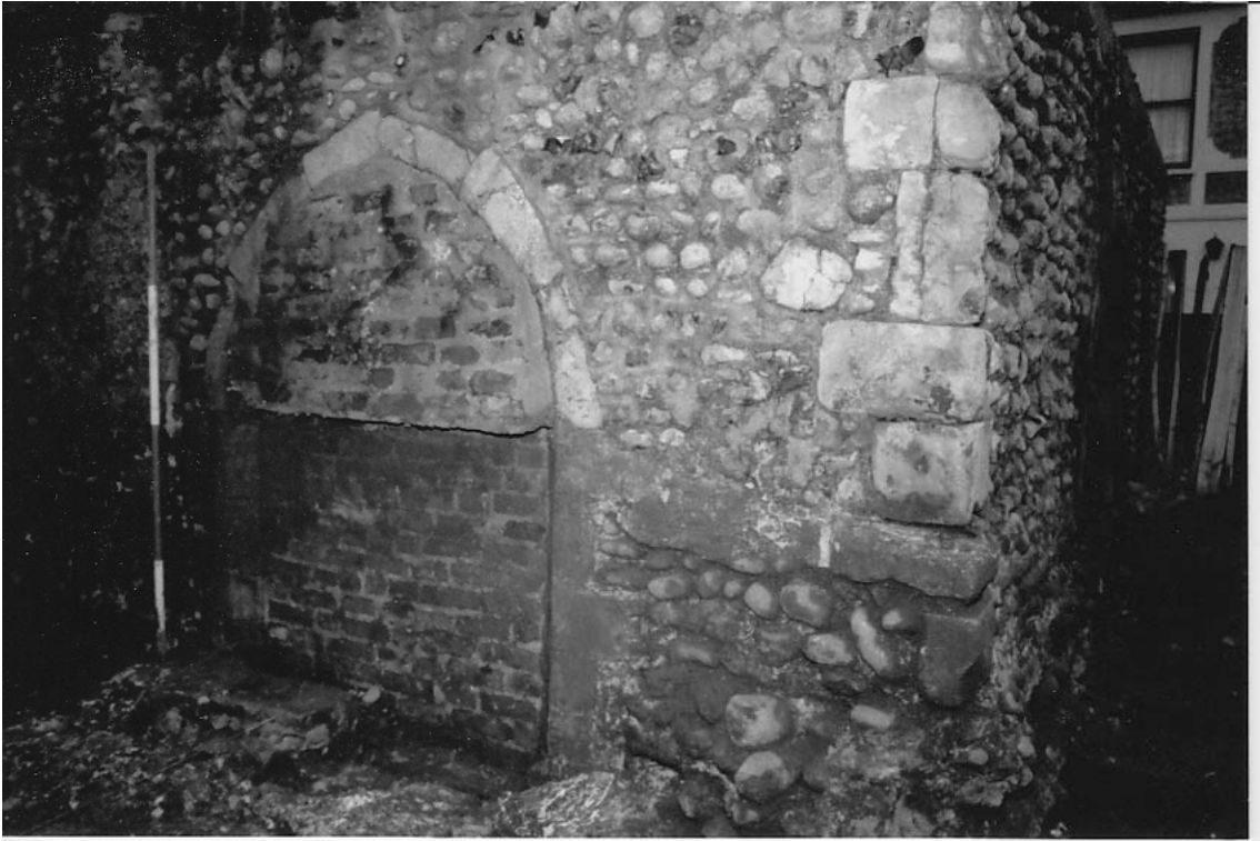
Main entrance, N wall [R557/30 - DM 1993]
