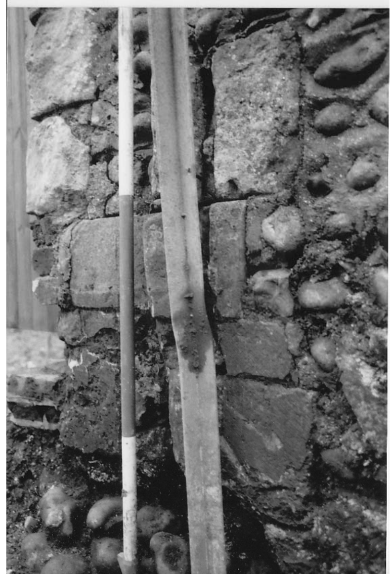
Door jamb at NE corner [R557/24 - DM 1993]
