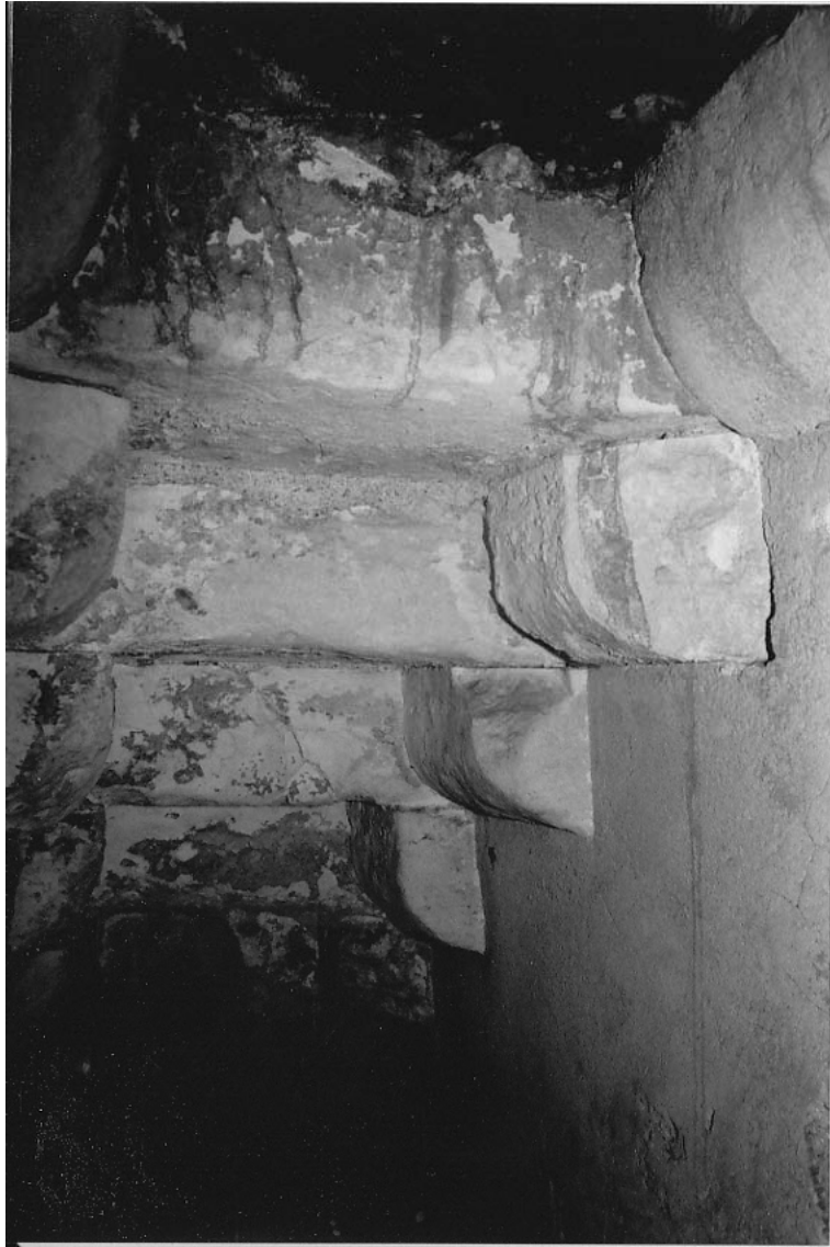
Roof of secondary stair [R557/17 - DM 1993]
