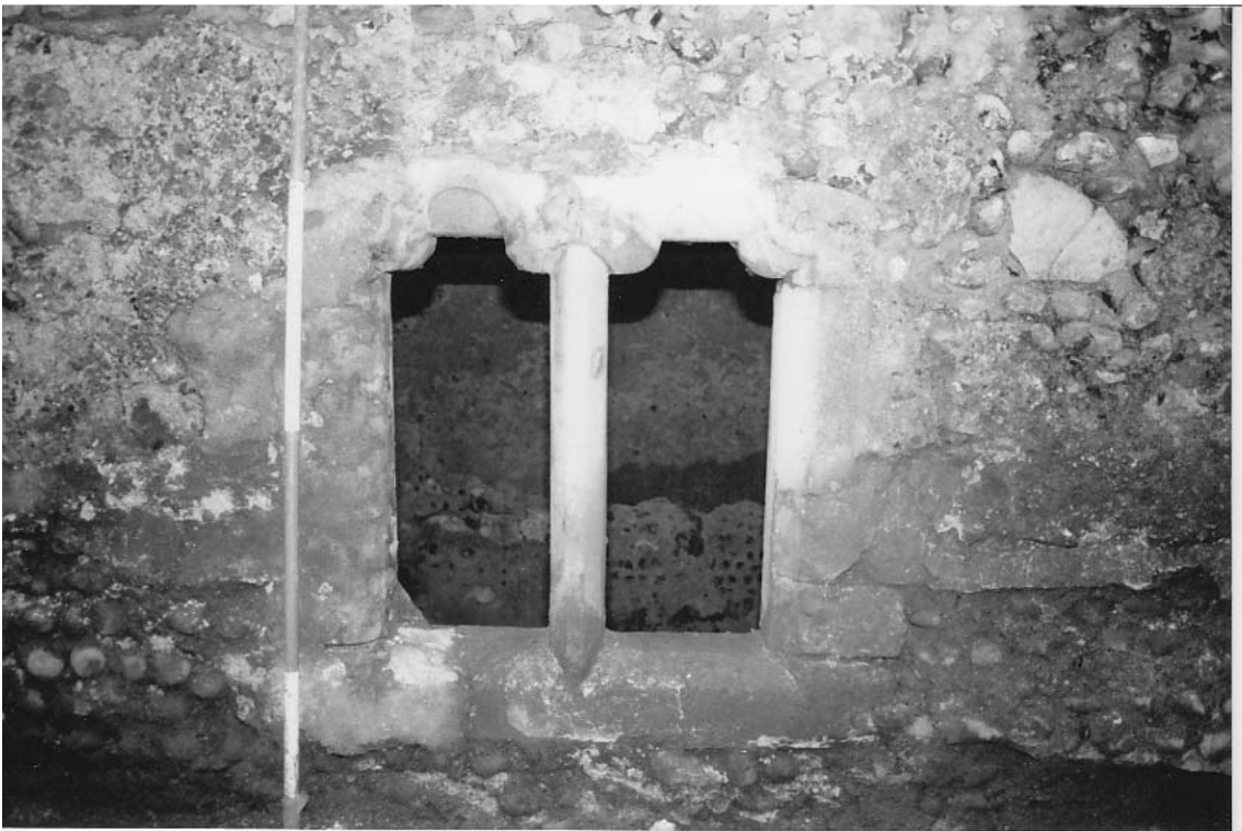
Window in N wall [R557/27 - DM 1993]
