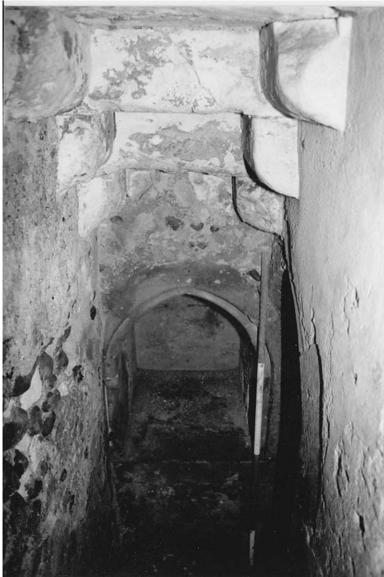
Looking down secondary stair [R557/15 - DM 1993]
