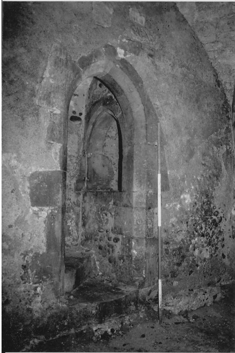
Door to secondary stair [R557/3 - DM 1993]
