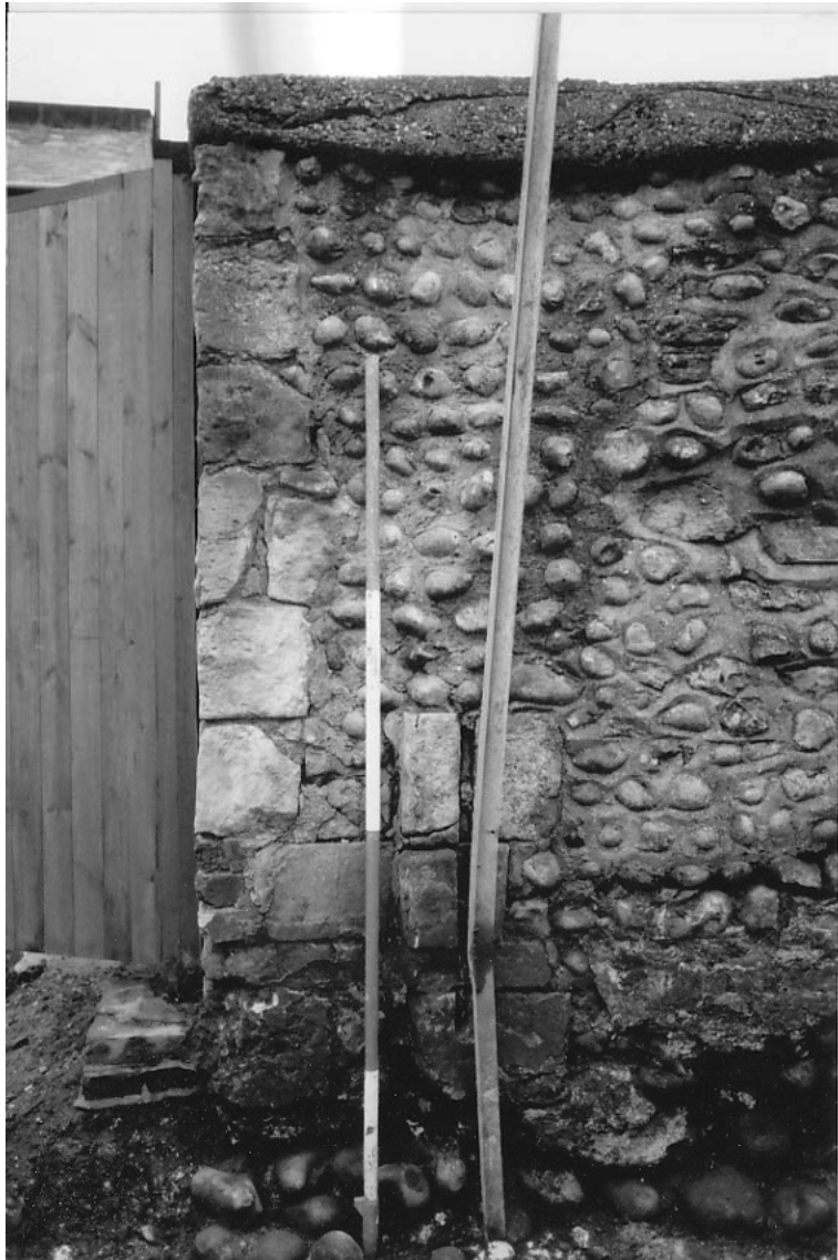
Door jamb at NE corner [R557/25 - DM 1993]
