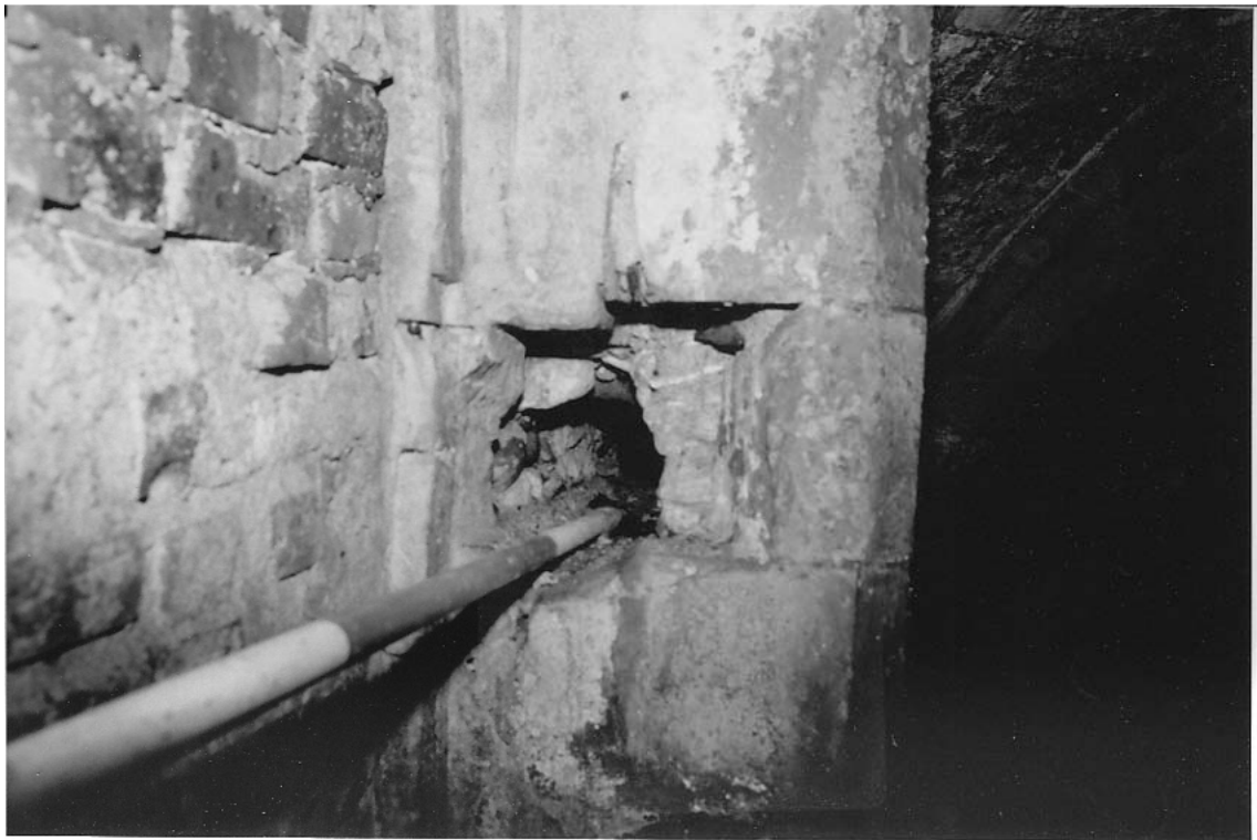
Locking point to main door [R557/20 - DM 1993]
