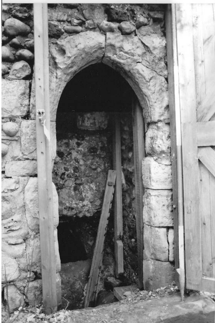
Entrance to secondary stair [R557/23 - DM 1993]
