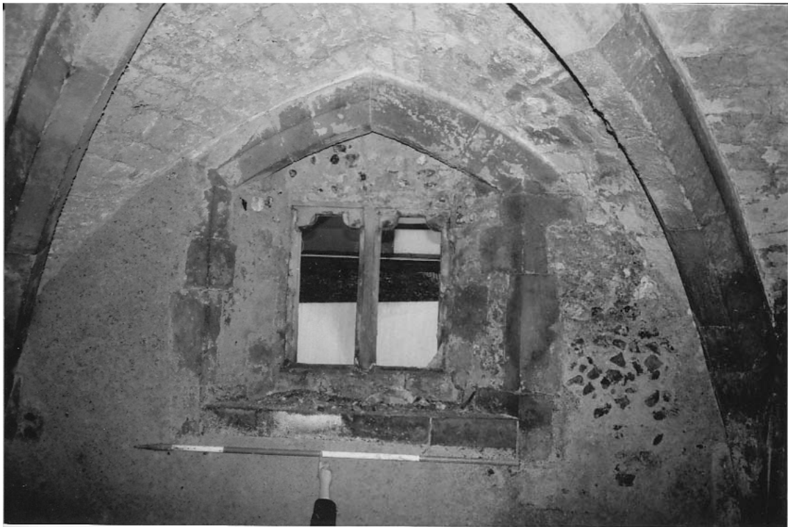
Window in north wall [R557/00 - DM 1993]
