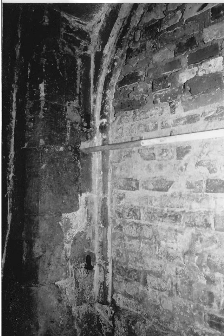
Pintles and locking point, main entrance [R557/21 - DM 1993]
